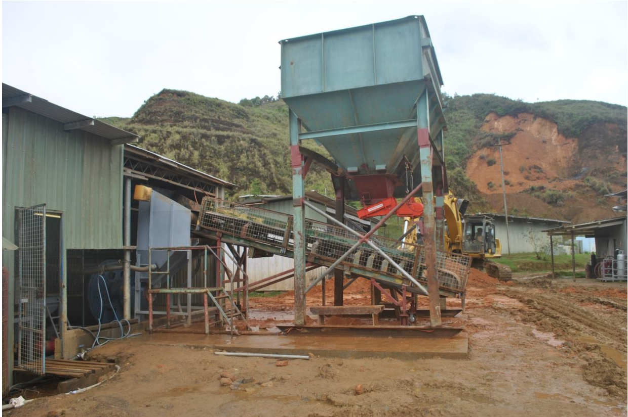
Testing and modifications are underway on the newly installed mechanical ball mill feeding plant
